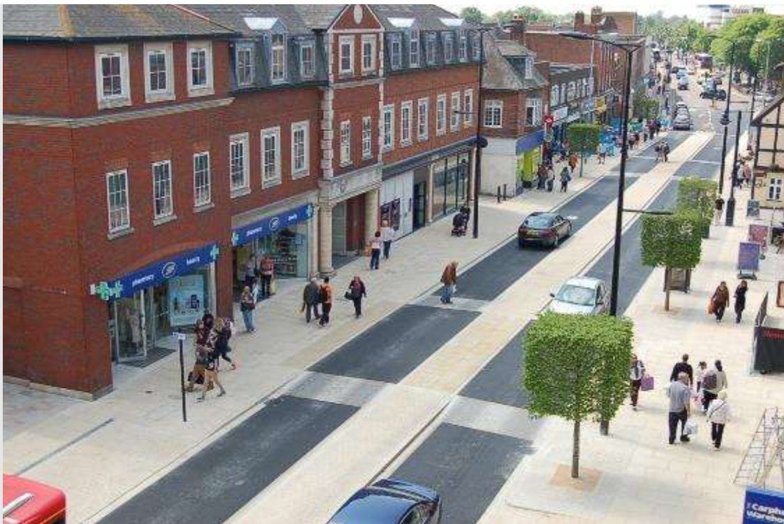
Figure 80 - Hornchurch Town Centre, Havering: A key feature of the scheme was a focus on improving pedestrian permeability. This was achieved by removing guardrails, placing crossings on desire lines, increasing the width of the footways and implementing a continual central pedestrian crossing strip. The scheme also improved social spaces through planting, new lighting, wayfinding and street furniture. Traffic flow was also improved, bus stops were made fully accessible, and better provision for cycling was installed.
