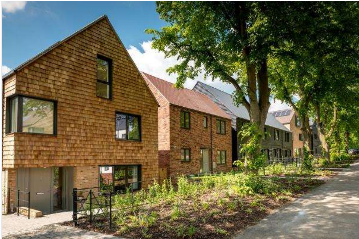
Figure 28 - The Avenue, Saffron Walden: Sympathetically designed to reflect the character of the surrounding area with a mixed palette of materials and crisp contemporary design detailing.
