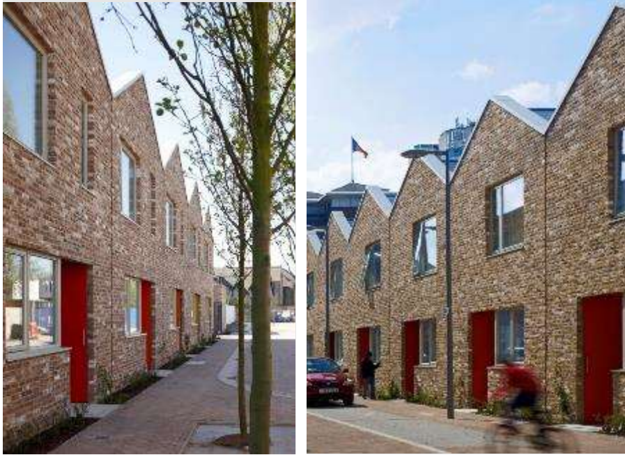
Figure 39 - Anne Mews, Barking: Traditional terraced houses focusing on the simple application of high quality materials and a generosity of scale, featuring large window openings, recessed entrances and integrated bin storage. The scheme creates a strong street frontage and a welcoming streetscape.
