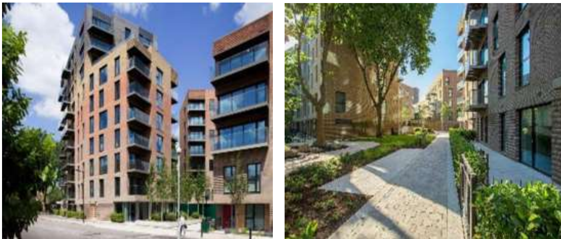
Figure 42 - Trafalgar Place, Southwark: Comprising of linear blocks, villa blocks and a tower, the scheme reconnects previously fractured surrounding neighbourhoods, creating a pedestrian link and an internal courtyard space. The design features simple building forms prioritising interior space and spaces between buildings. Different shades of brickwork are used to define key elements giving each building a slightly different character.
