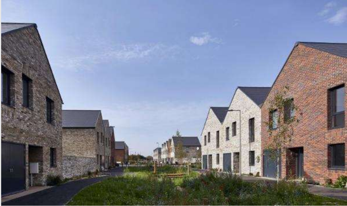
Figure 26 - St Chad's, Tilbury: Traditional pitched roof forms with high quality materials and detailing create a familiar but contemporary feel.
