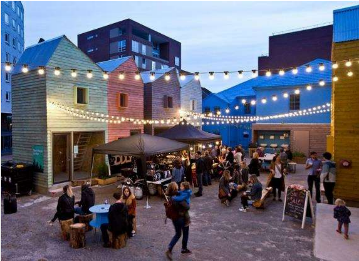
Figure 47 - Blue House Yard, Haringey: A redevelopment and re-imagining of a disused car park site, the project combined creative maker space with public space, creating retail and workspace opportunities bringing activity and life to the yard throughout the day and evening.
