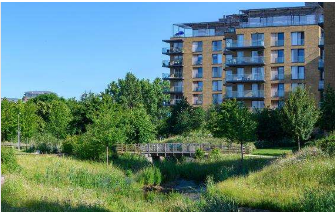
Figure 66 - Cator Park, Kidbrooke Village, Greenwich: Working in collaboration with the London Wildlife Trust a landscape-led approach supports the green infrastructure network beyond the site boundaries providing flood mitigation measures and water management. The high quality biodiverse parkland provides a natural setting for the development supplemented by a range of private and semi-private amenity spaces.
