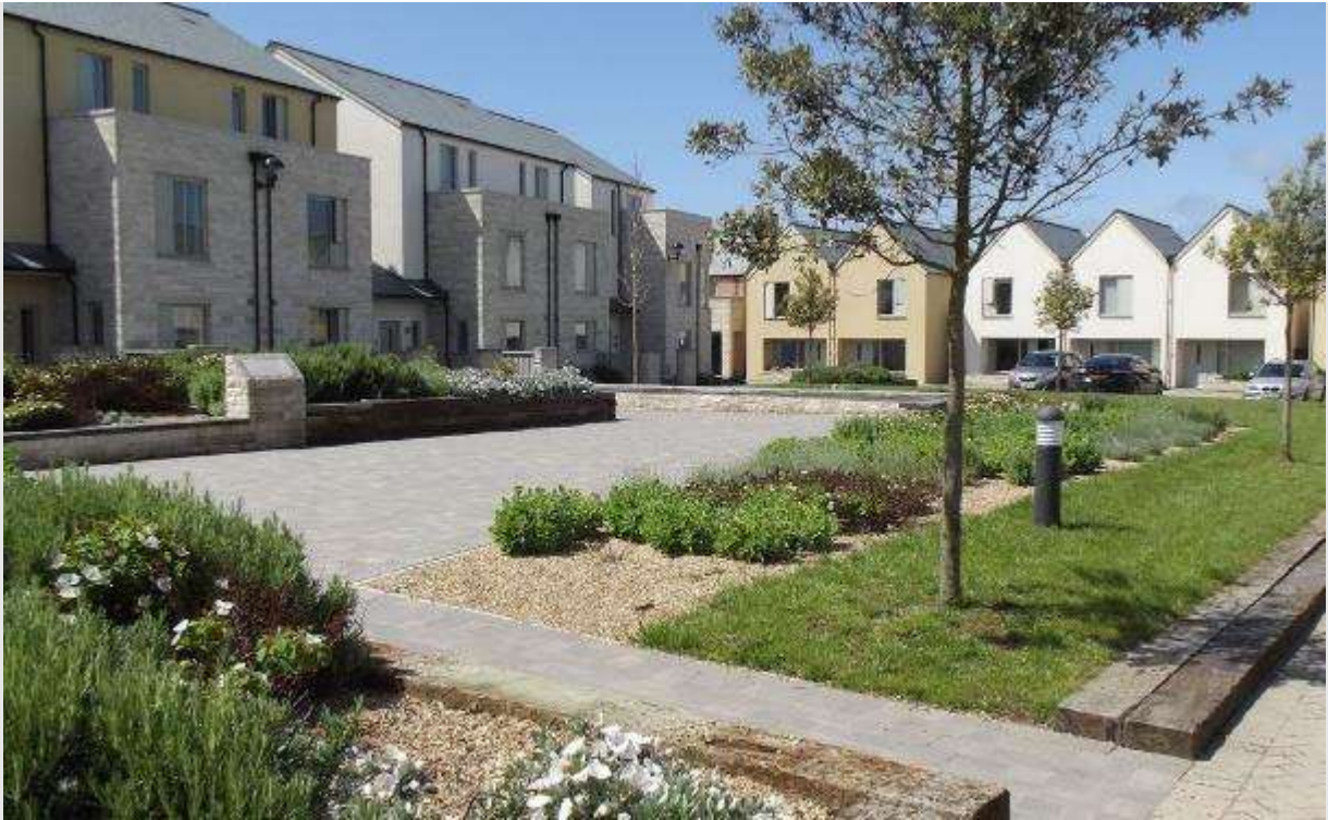
Figure 88 - Officers Field, Weymouth: Prioritising sustainable living through a fabric-first approach and a mix of home sizes and tenures each with access to private and shared open space. Benefiting from light and space the homes feature a highly insulated fabric with energy generated by an on-site biomass CHP system and PV panels.
