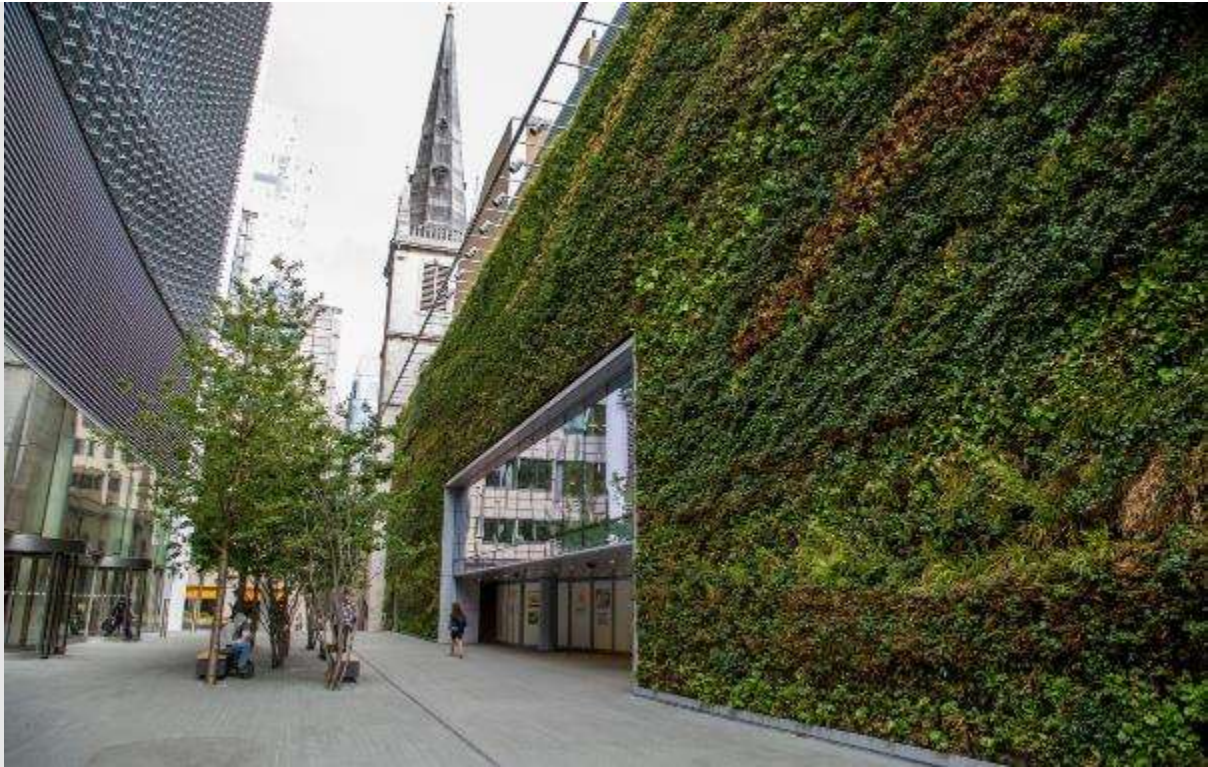
Figure 96 - Fenchurch Street, London: At over 700sqm this living wall contains around 52,000 plants. The wall was installed on an annex service building opposite the southern entrance providing visual amenity with urban climate mitigation and biodiversity benefits.
