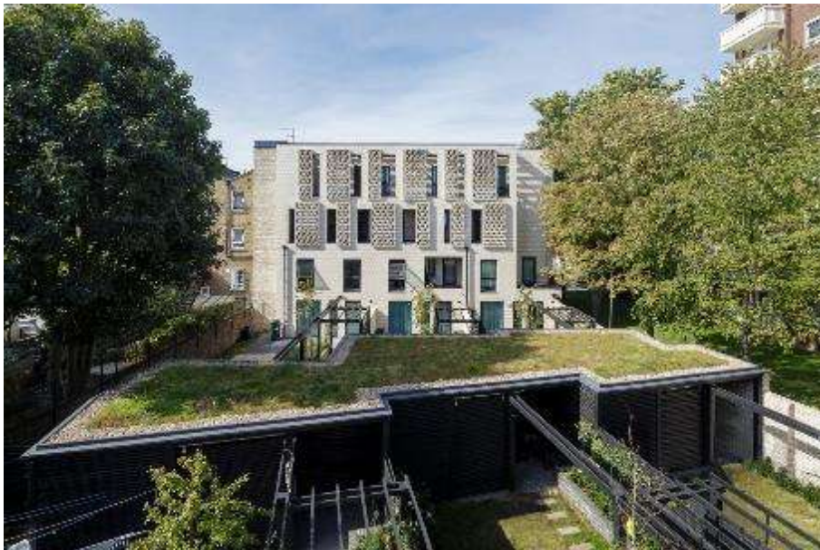
Figure 43 - Vaudeville Court, Islington: The design features a mix of maisonettes on the ground and first floors, and two-bedroom flats above. Arranged in two terraces, with private gardens between them, the scheme references the scale of neighbouring buildings and reinstates the street frontage. The family homes are dual aspect with open plan living space and a private courtyard garden. Garden rooms give families extra amenity and storage space.
