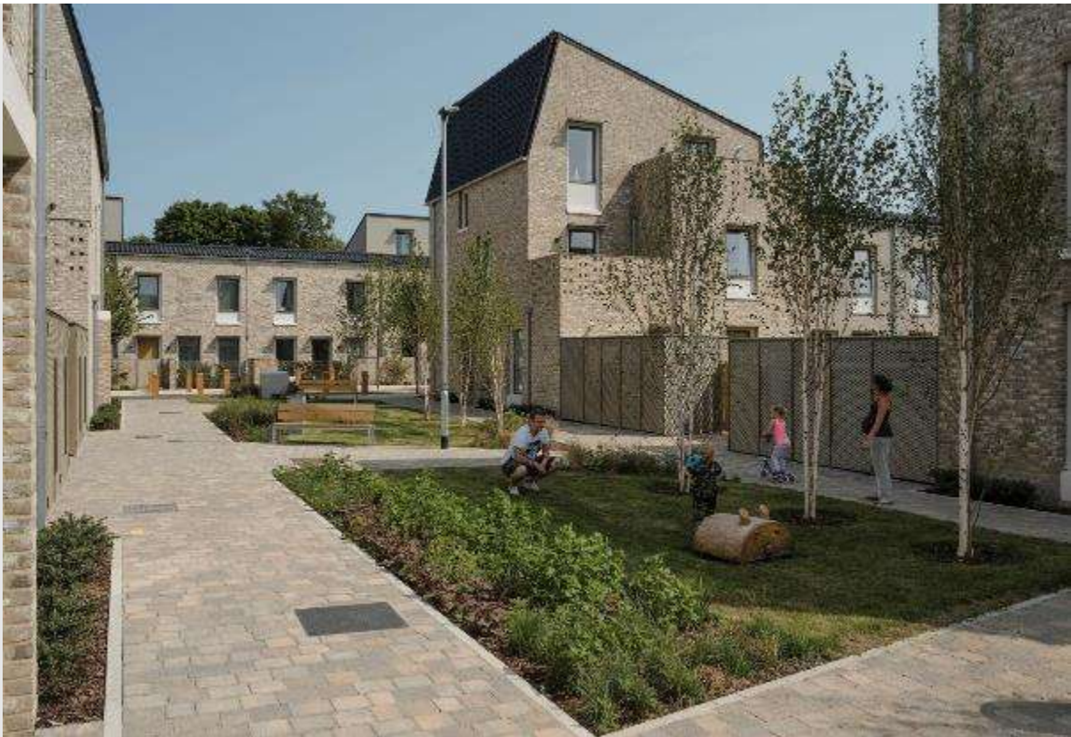
Figure 13 - Goldsmith Street, Norwich: A fine grain street based approach in response to the surrounding context; a series of terrace blocks with reduced distances between properties (14 metres) creates a low-rise, high-density development with strong frontages and neatly framed communal amenity spaces.
