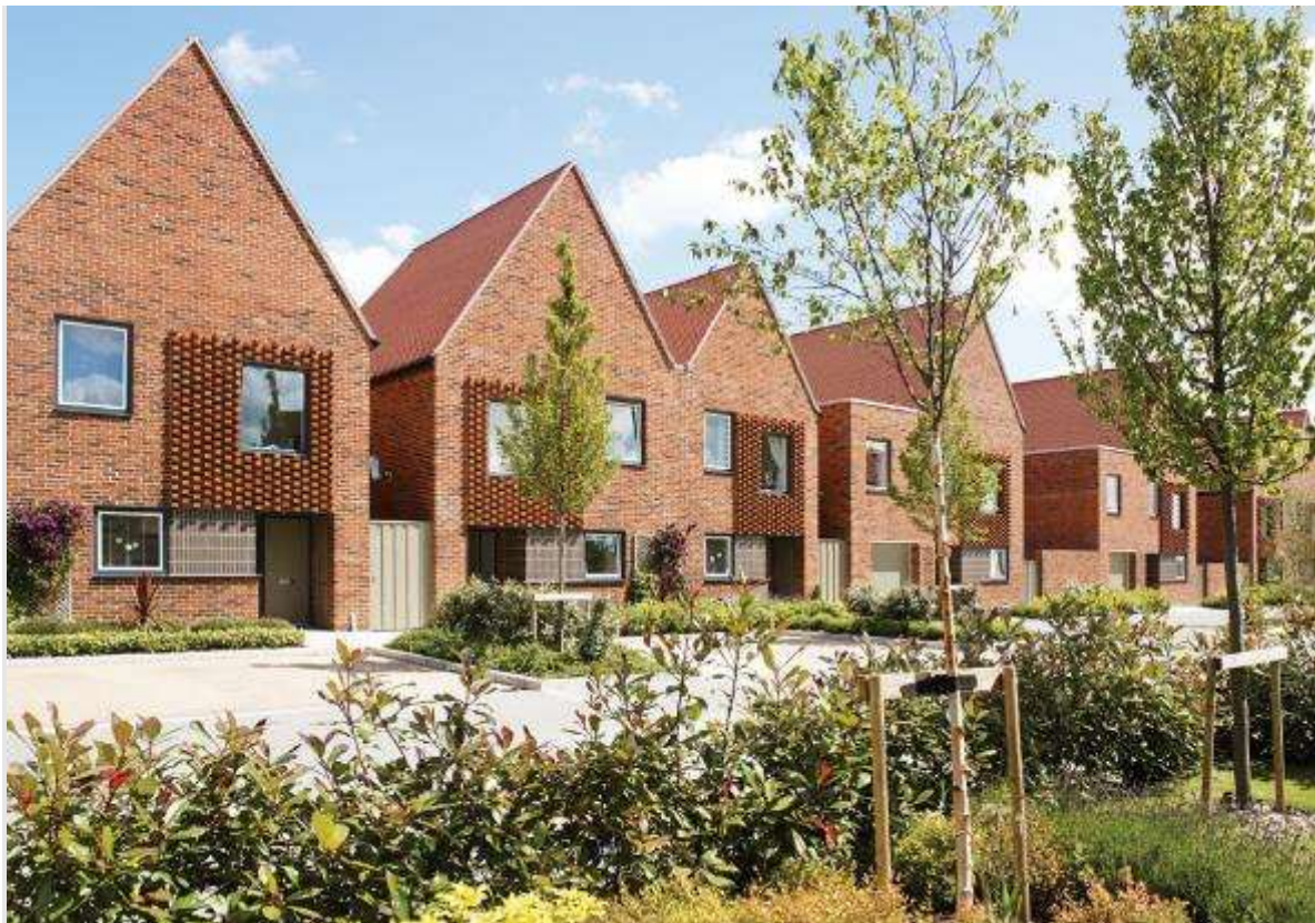
Figure 38 - Horsted Park, Chatham: Pairs of semi-detached houses with recessed entrances and expressed gables provide a strong rhythm to the streetscape. Projecting chequerboard brickwork patterning provides a visual identity and sense of character.
