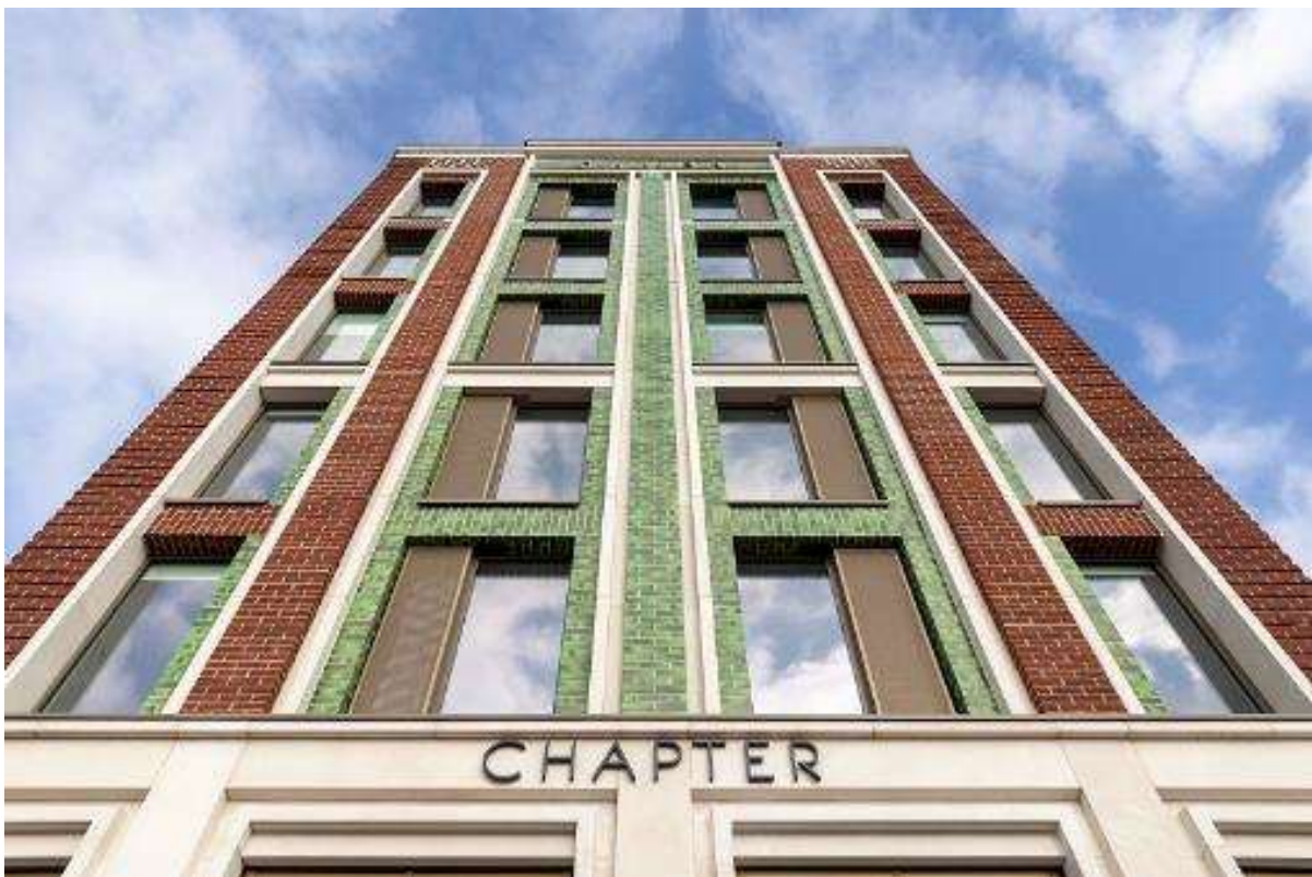
Figure 16 - Savoy Circus, Wembley, Brent: Influenced by the local context, architectural details include corbelled brick corners, reconstituted stone window surrounds and glazed brickwork providing articulation and visual interest to break up the massing of the building. The design sits sympathetically within a Conservation Area setting.
