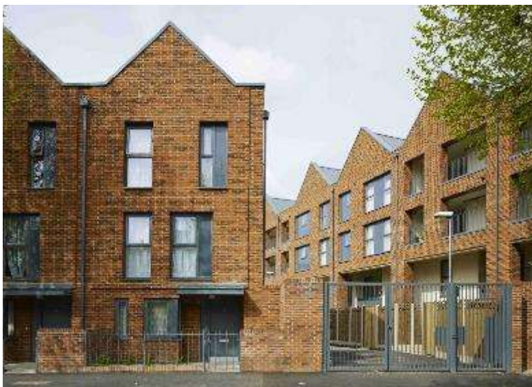
Figure 40 - Hammond Court, Waltham Forest: Carefully crafted architecture with an emphasis on quality of place; terraced houses, maisonettes and flats enclose a south facing courtyard with shared and private amenity spaces. Homes are dual aspect with generous space standards designed for longevity and flexibility.
