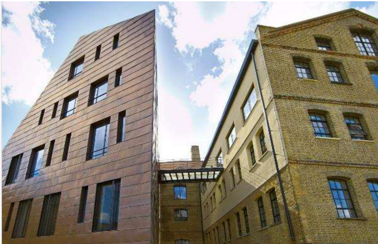
Figure 30 - The Granary, Barking: A new bronze clad extension takes its cue from the gabled form of the original building and is attached via the vertical circulation core and a high level bridge link. The contemporary design clearly distinguishes the 'old' from the 'new' whilst respecting the existing 19th Century building.
