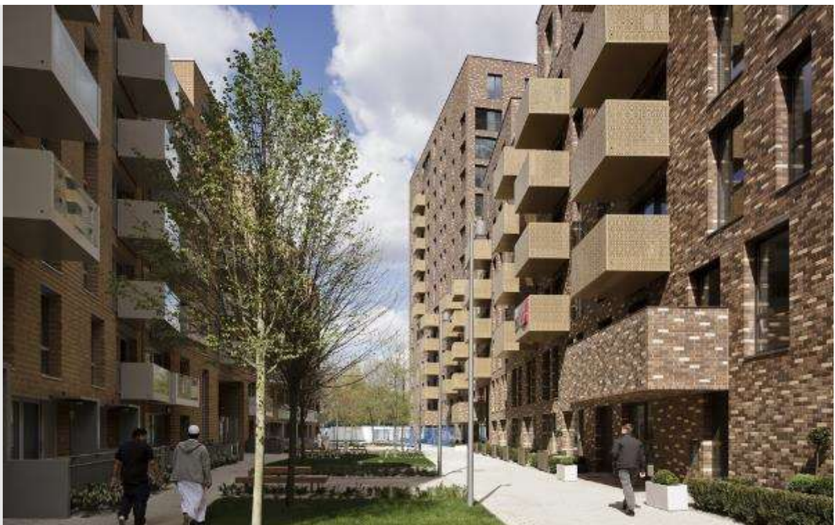
Figure 15 - St Andrews, Bromley-by-Bow: Brickwork facades with a rich mix of bonds and colours, deep window reveals, generous balconies, and a variation in storey heights break up the scale of the blocks which form part of a high density residential-led scheme.
