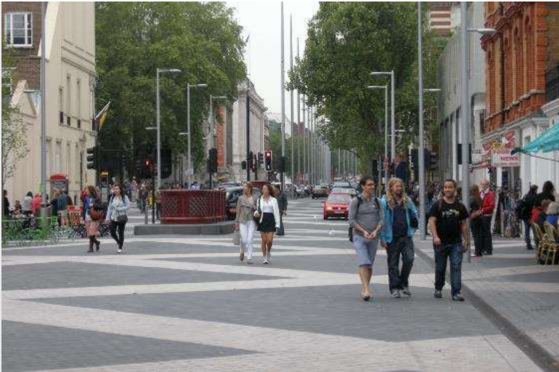
Figure 79 - Exhibition Road, Kensington: A shared surface approach with a single level surface from building face to building face along the entire length of the road. Within this single surface the needs of the pedestrian, cyclist, motorcyclist, car, taxi, delivery vehicle, and bus have been carefully considered. Changes were made to the surrounding road network to reduce through traffic and enable mixing of pedestrians cyclists and vehicles. The diagonal paving pattern reflects the movement of people from one side of the street to the other.
