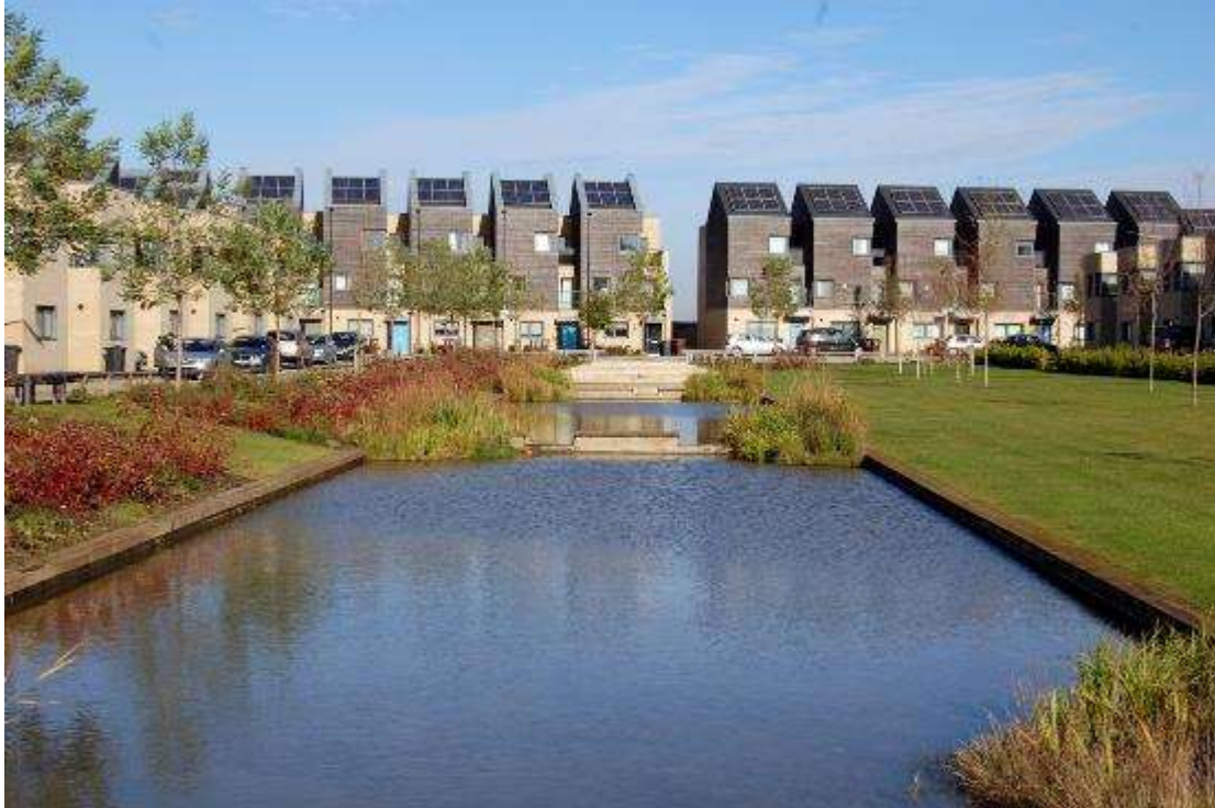
Figure 94 - Barking Riverside, East London: A 179 hectare brownfield site situated on the north bank of the River Thames with planning permission granted for over 10,000 homes. Over 40% of land is dedicated to open space including parkland linked by cycle routes and footpaths. A range of environmental measures include energy saving homes, rainwater harvesting, SUDs, green roofs, and conservation of local biodiversity.
