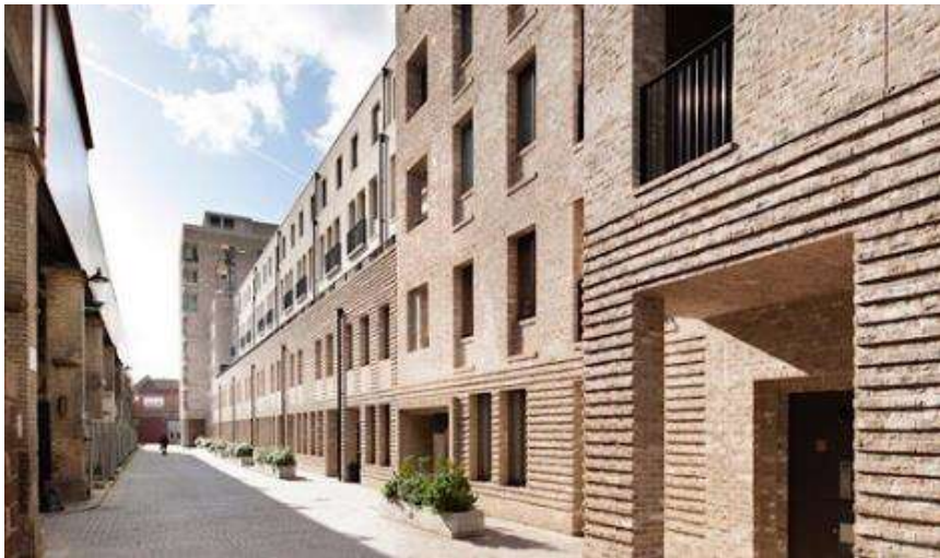
Figure 41 - Silchester Estate, Kensington and Chelsea: A mix of housing typologies combined to create a legible human scale urban block enclosing a shared garden. Openings have a vertical emphasis with regular repeated proportions creating a rhythm to the streetscene. All homes are dual aspect providing good levels of daylight and cross-ventilation with access to private amenity space.
