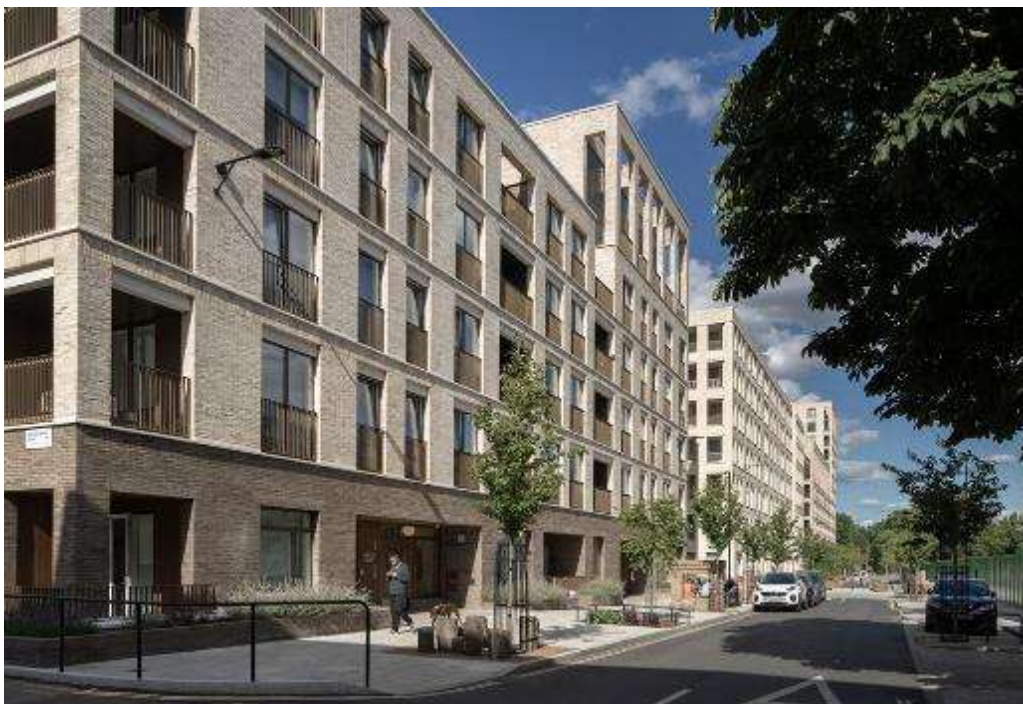
Figure 83 - Kings Crescent Estate Phases 1 & 2, Hackney: A local authority-led development involving intensive consultation with residents and local people who helped to define all aspects of the scheme including the planning of streets, internal layouts and material specifications. Three courtyard buildings combine existing and new blocks with shared amenity spaces and dual aspect entrance lobbies featuring the same level of design quality regardless of tenure.
