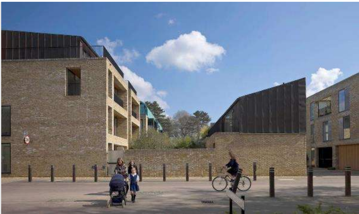
Figure 27 - Accordia, Cambridge: Adapting a traditional housing typology with a distinctive asymmetrical roof form, optimising light, ventilation, and internal connectivity whilst maintaining a terrace-like urban form to the street.
