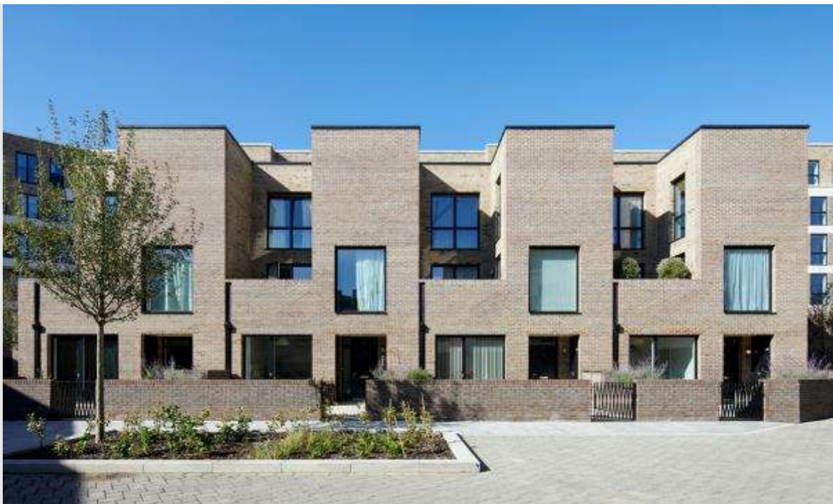
Figure 31 - Park View Mansions, Chobham Manor: Generously sized openings help to break up the mass of the three-storey townhouses, the positioning adds rhythm to the facade animating the elevation
