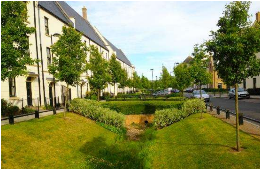
Figure 95 - Upton, Northampton: Sustainable Urban Drainage Systems are incorporated throughout the masterplan (an urban extension of approximately 1350 homes) with generously sized swales contributing to the character, identity and biodiversity of the neighbourhood. The swales have both functional and aesthetic benefits; reducing flood risk by storing and infiltrating water runoff, whilst also creating attractive green corridors which soften the streets.
