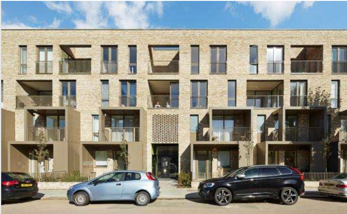
Figure 32 - Ely Court, Brent: A rhythmic composition of recessed windows, front porticoes, upper porticos and recessed balconies creates a highly articulated street facade.
