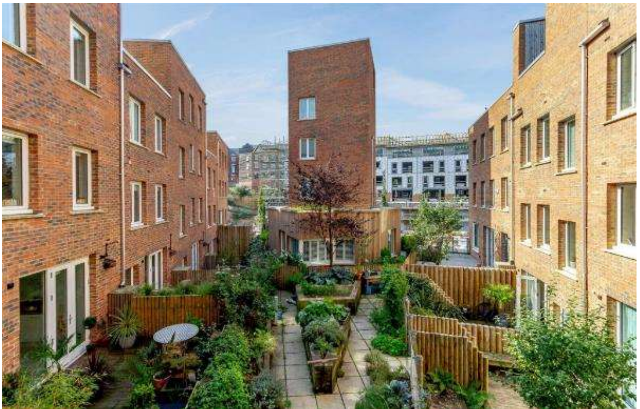
Figure 12 - The Malings, Ouseburn: An alternative street-based approach to conventional flatted blocks. New streets run down a sloping site towards the river, optimising views and following desire lines to connect surrounding neighbourhoods. The Malings blends traditional street typologies with a combination of courtyard dwellings, back-to-backs, and taller townhouses.
