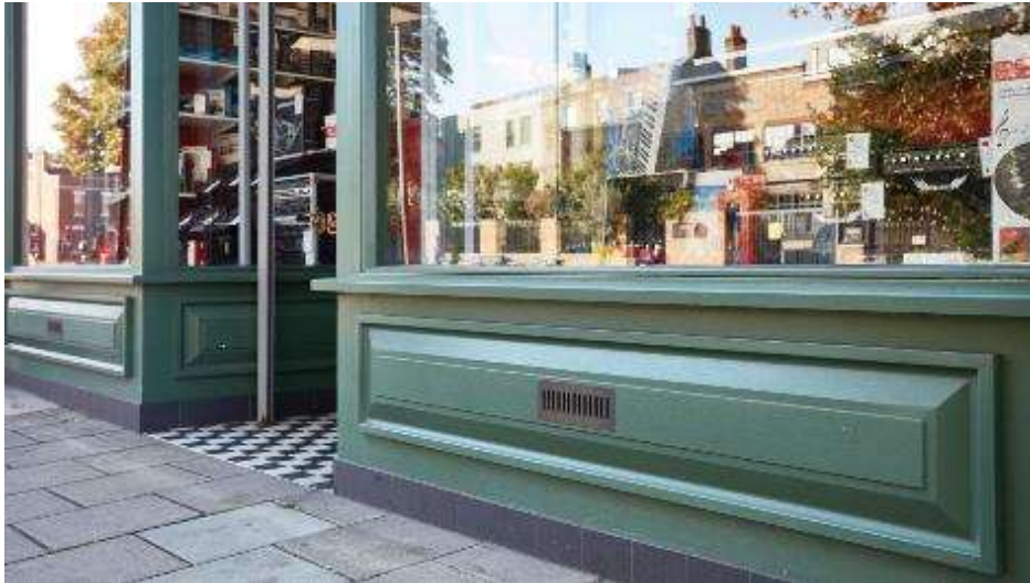
Figure 56 - A traditional shopfront stallriser
