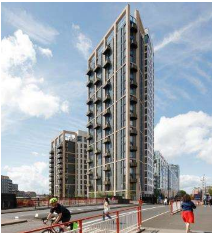
Figure 93 - Union Wharf, Greenwich: One of the first high-rise residential projects in the UK to use volumetric off-site construction; although initially designed to be delivered traditionally, the rationalisation of design elements and a repeated floorplate enabled its conversion to modular build construction, retaining design quality while maximising the benefits of off-site design and delivery.
