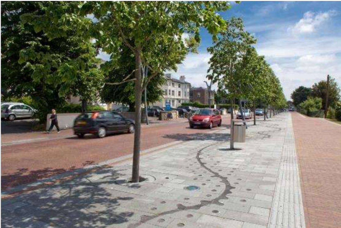
Figure 81 - Elwick Road, Ashford: The transformation of an existing one-way three-lane road, applying a shared space philosophy, into a two-way street. The scheme creates a more permeable link from the station and town centre to a southern expansion area. The paving design references the Stour River, it provides a 'natural' demarcation between the vehicular and pedestrian zones and creates a visual and functional link that ties the town centre to the station and further afield to the river.
